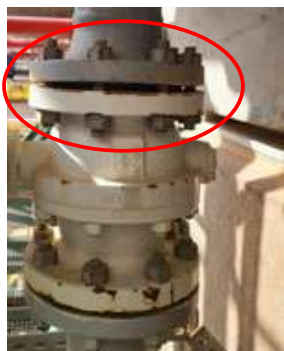
Fig. 2 The flange at the lower nozzle F1 (4") was found distorted, but leaking has not been observed while the vessel was in service
